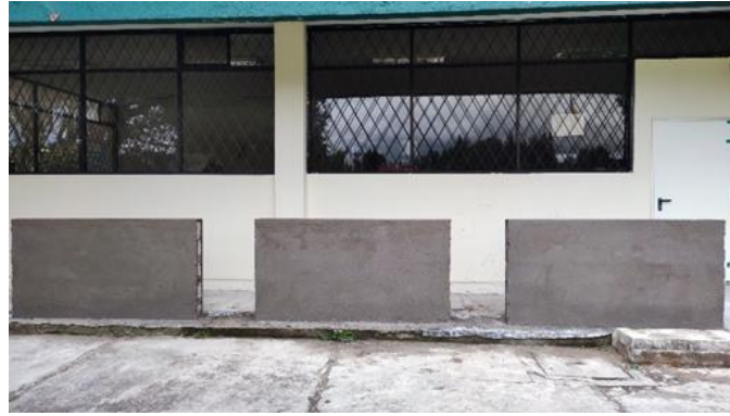
Fig. 15. Plastered Pressed Block Masonry
