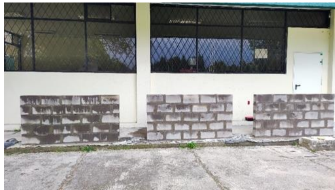
Fig. 14. Pressed block masonry
