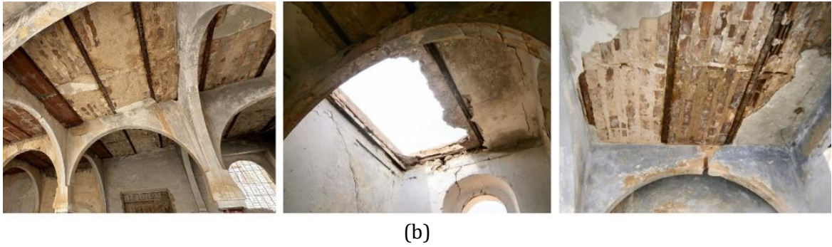
Fig. 7. Views of the roof structures in the ksar of Lichana: palm wood post-and-beam; b) IPN joists of the mosque. Photos by authors, 2024
