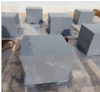
Fig. 5. Application of epoxy
