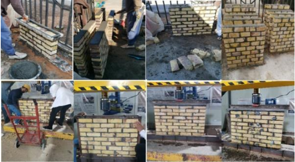
Fig. 4. Construction and setup of walls to test
