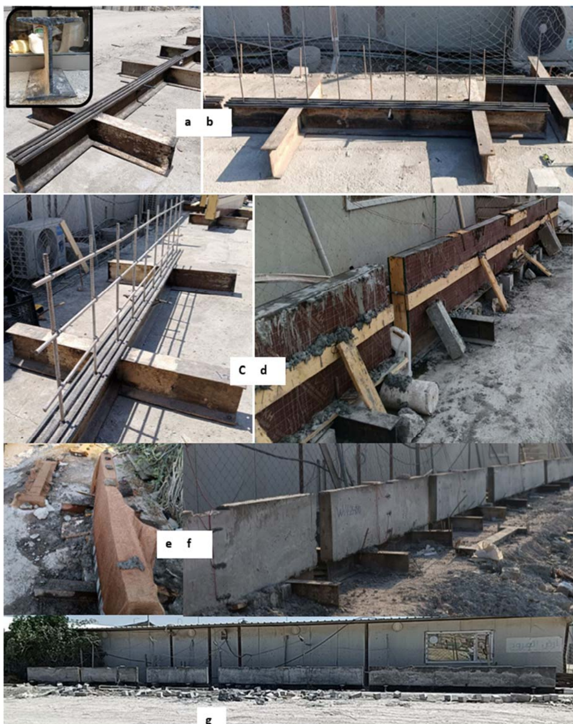
Fig. 2. (a), (b), (c) preparing walls, (d) casting, (e) curing, (f) strain installation., (g) The five hardened walls
