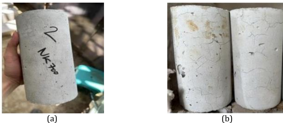
Fig. 13. Physical condition of normal concrete specimens before and after exposure to 700°C: (a) before burning, bright gray in color; (b) after burning, showing no significant color change, with increased localized yellowish spots, longer cracks, and spalling
