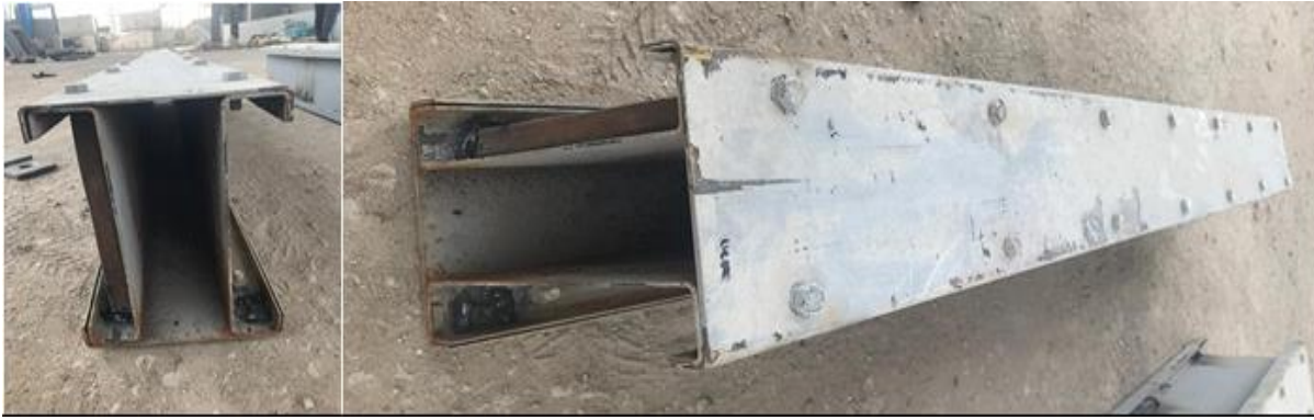
Fig 13. Failure Mode of Beam BH0.7
