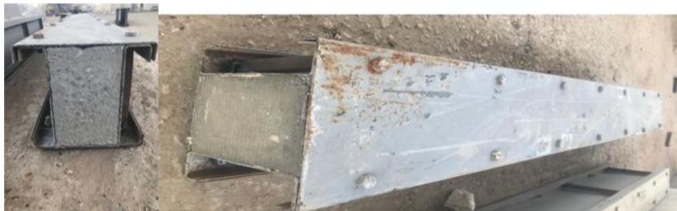
Fig. 20. Failure mode of beam BC1.3
