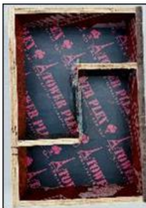
Fig. 2. Preparation of plywood formwork and reinforcement
