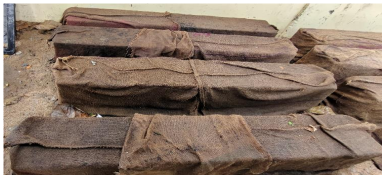
Fig. 5. Membrane curing of R.C.C Beams
