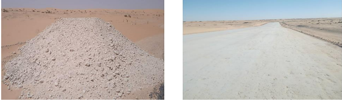
Fig. 1. Gypseous-calcareous soil before and after compaction
