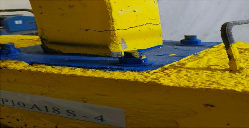
Fig. 22. Failure mode of (4 P10 A18 S -4) specimen
