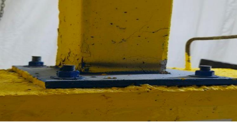
Fig. 23. Failure mode of (4 P15 A16 S -4) specimen
