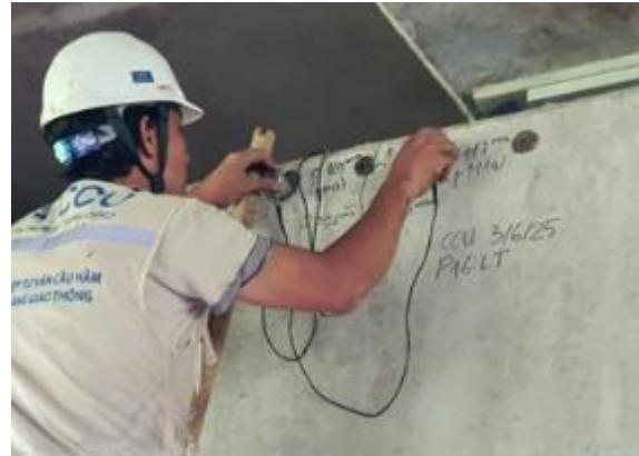
(b) Measurement of crack depth using ultrasonic tester (C369N)
