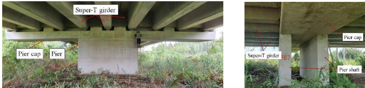
(a) Overview of investigated pier
