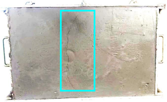
(d) Appearance of Full Crack after 12 hours
