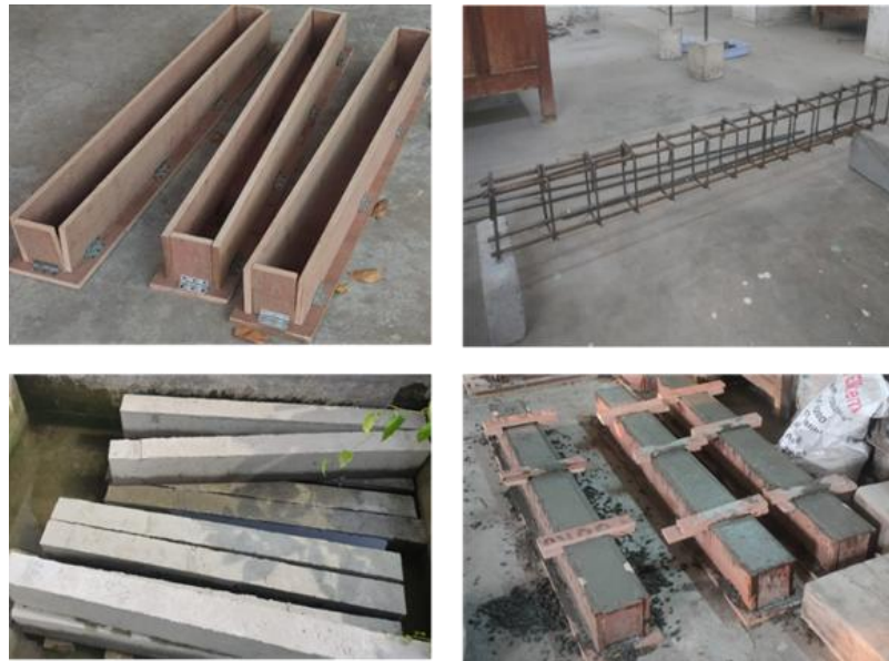
Fig. 1. Experimental setup for casting concrete beams
