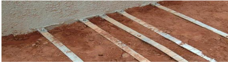
Figure5. How to fix aluminum strips ends in the field to prevent
