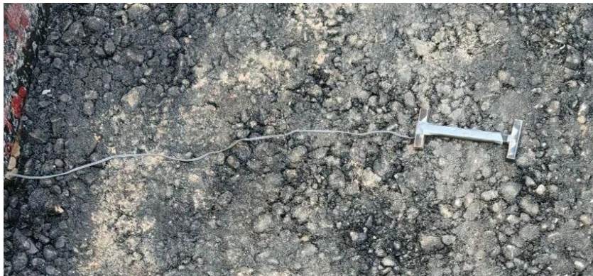
Fig. 5. Installation of asphalt strain gauges for tensile strain monitoring
