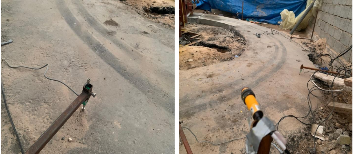
Fig. 6. Installation of Linear Variable Differential Transformers (LVDTs) for rut depth measurement
