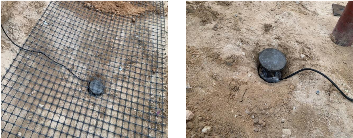
Fig. 4. Installation of the subgrade load cell used for vertical stress measurement
