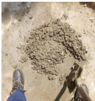
(a) Batching and mixing
