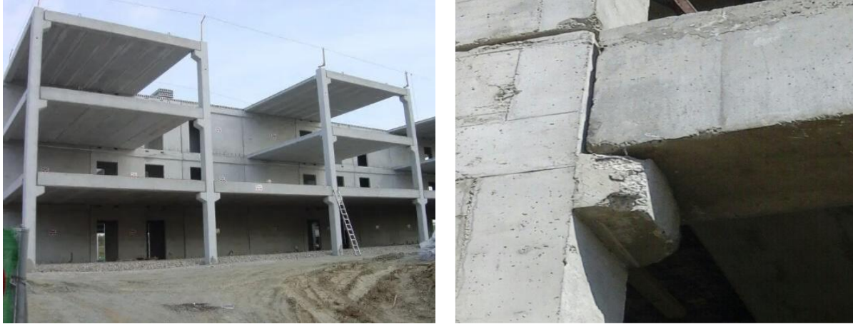
Fig. 1. Some types of corbels in buildings [15, 16]
