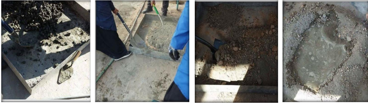
Fig. 6. Preparation and mixing of concrete stages
