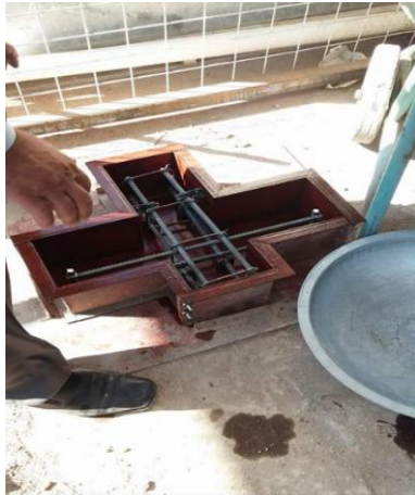
Fig. 7. Steel reinforcement within the framework
