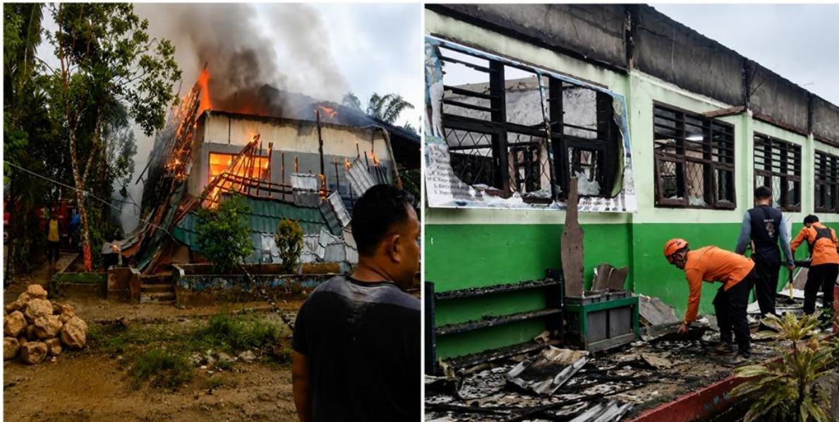
Fig. 1. Field documentation of the fire at SDN 022 Penajam (31 January 2024), which motivated the present experimental investigation. The left photograph shows the building during the active fire, while the right photograph shows the post-fire condition after fire suppression, including extensive fire damage and debris clearance prior to structural assessment. Photos: Field documentation by the authors
