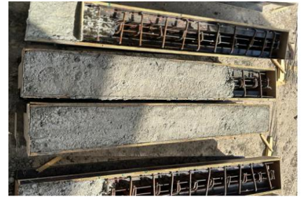
(f) Staged casting showing exposed reinforcement before subsequent placement
