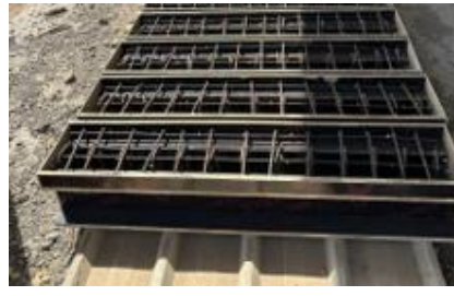
(b) Reinforcement cages before concrete placement
