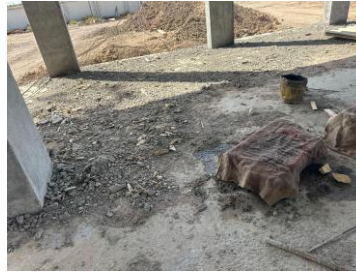
(d) Wet-burlap covering used for moist curing
